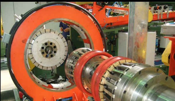
2nd Stage TBM Upgrade - Tooling
